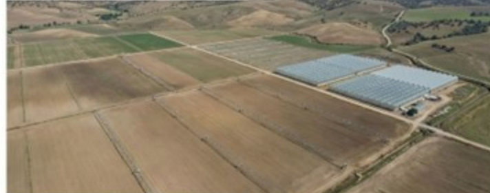
EPC EXECUTION - MIXED TERRAIN
